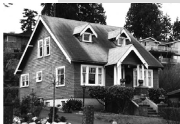
The intersecting dormers and porch gable provide visual interest to this otherwise unbroken roof plane.
