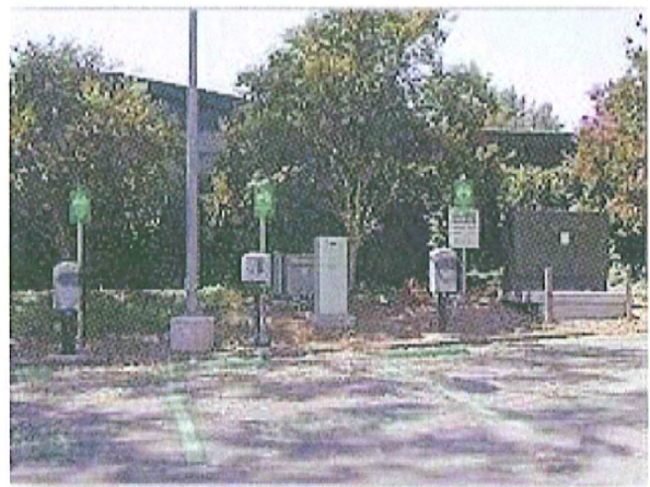
A typical Level 2 pedestal-style charging station in a surface parking lot. Photo courtesy of ECOtality.
