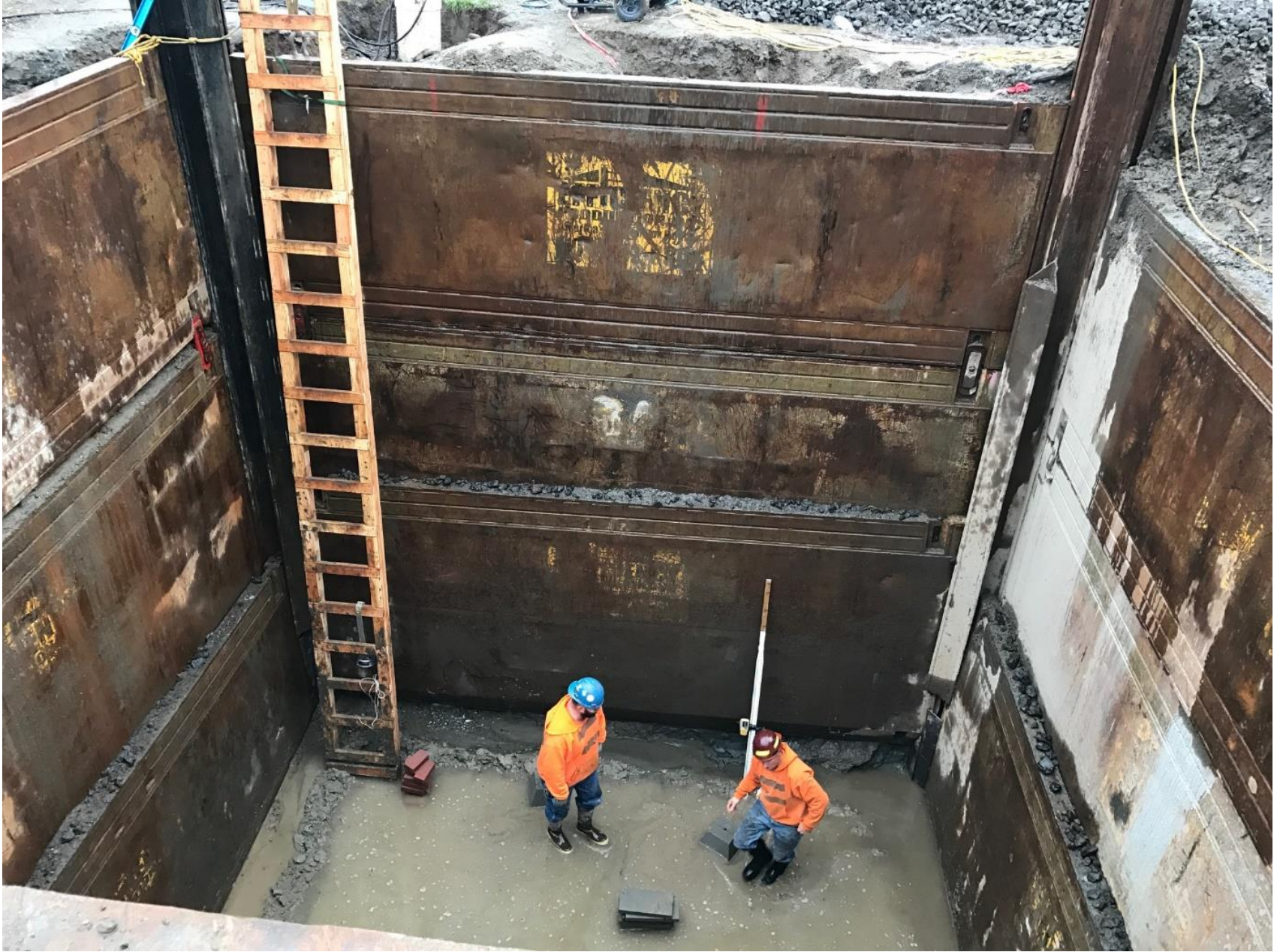
WET WELL EXCAVATION
