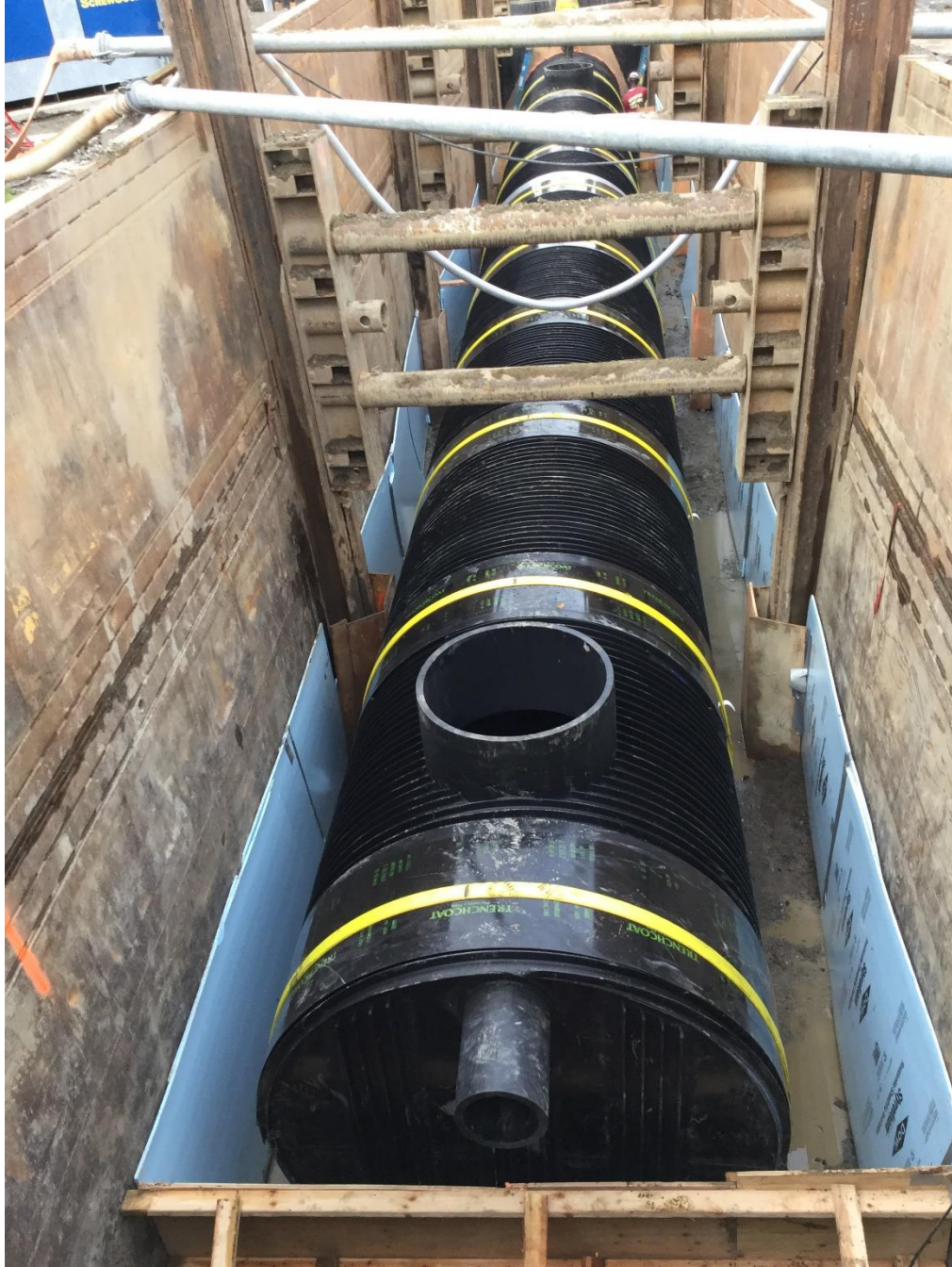
STORAGE PIPE INSTALLATION
