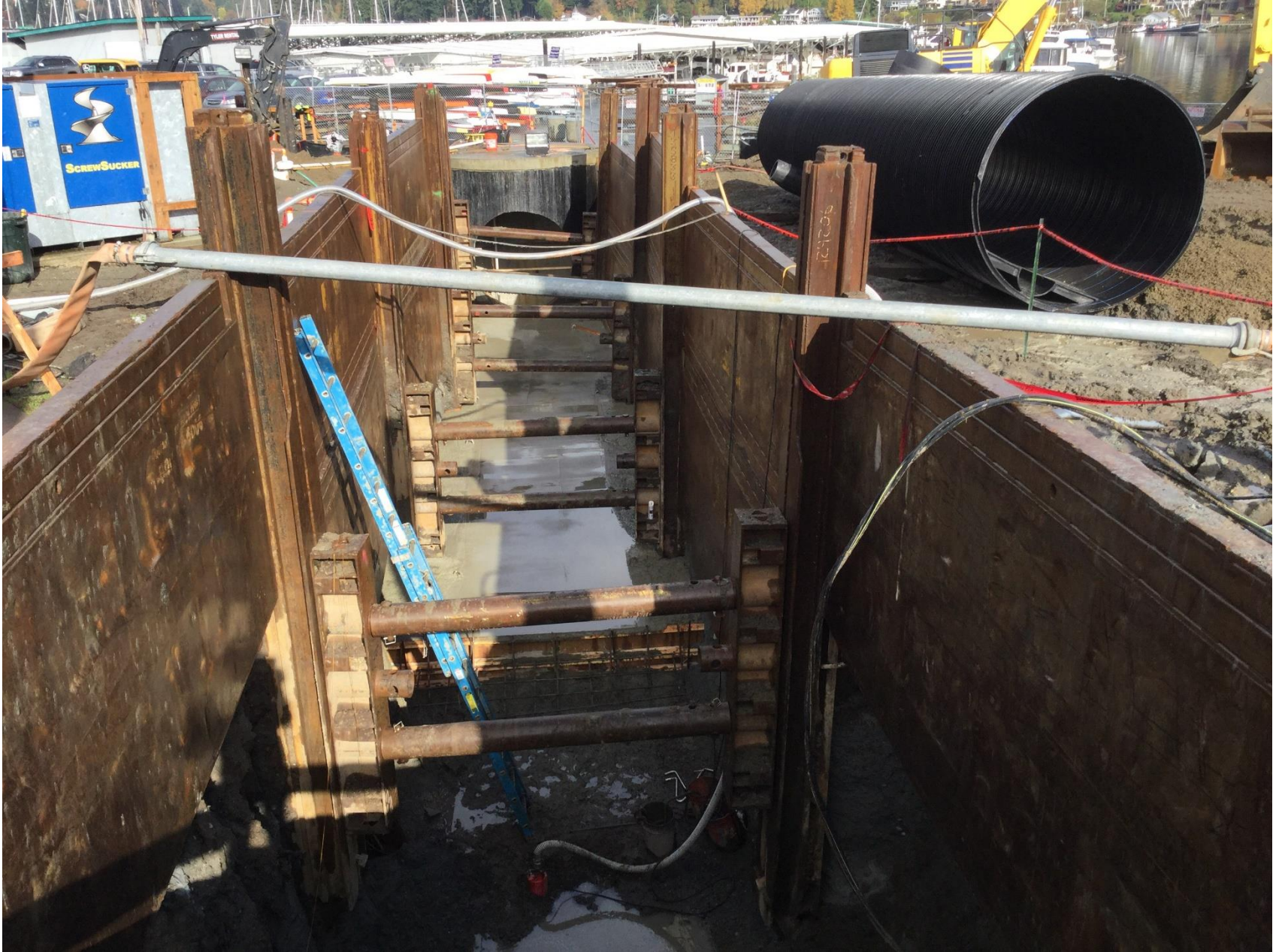
STORAGE PIPE EXCAVATION
