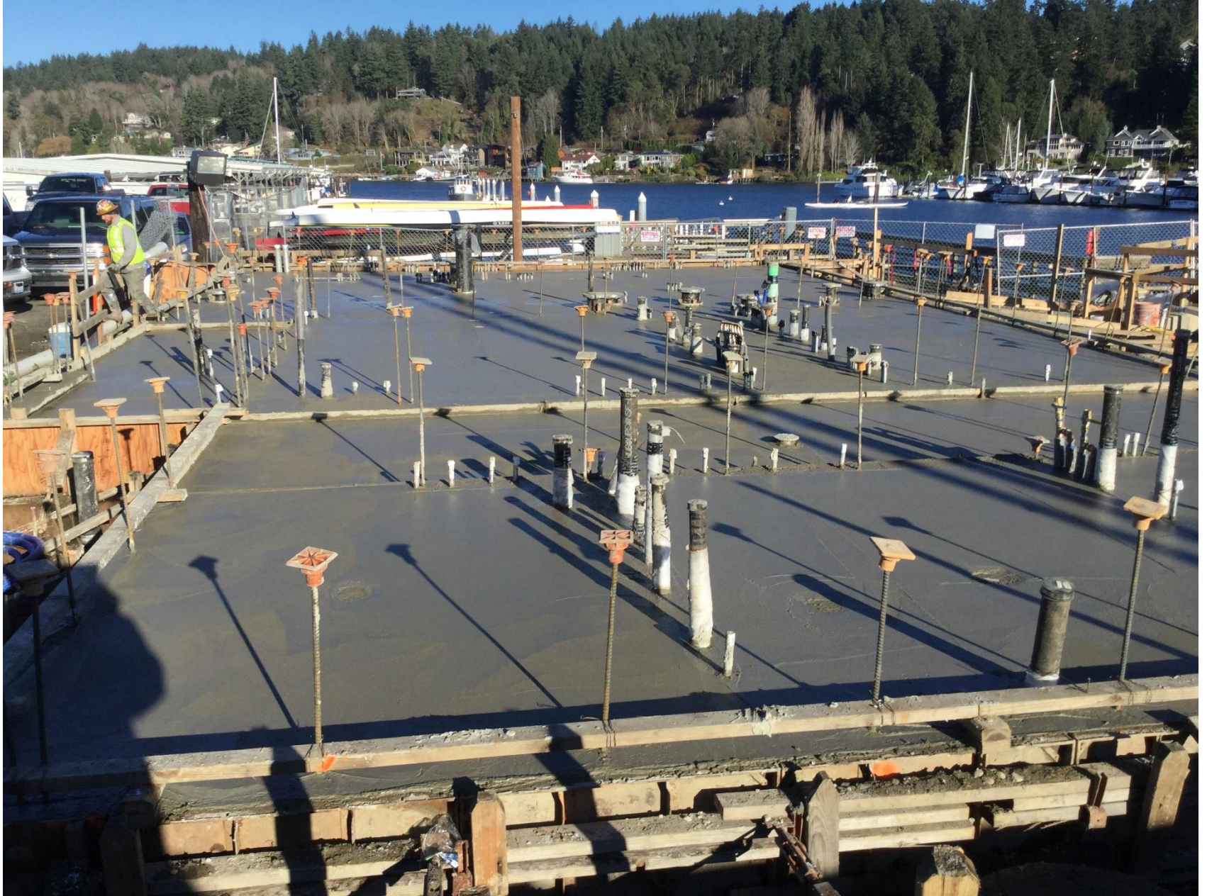
POURED BUILDING FOUNDATION
